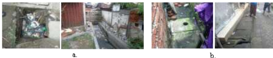
Figure 5. a. Drainage have sedimentation and covered by garbage; b. Utilizing the drainage as a sanitation disposal site mixed with domestic waste (Source: photograph by author,2017)
